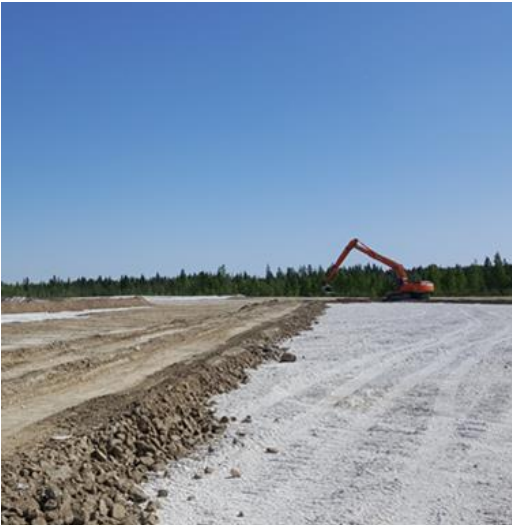
Full scale pilot construction (Best material for structure)
